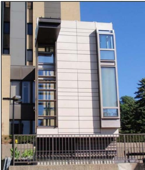
**Figure 2** Mock Up of the Terra Cotta Tile System
