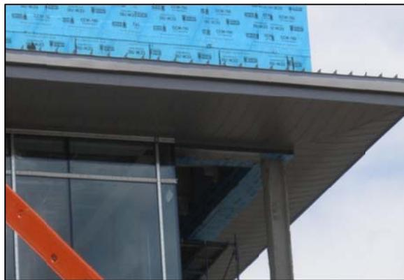
**Figure 1** Aluminum Cladded Eyebrow
